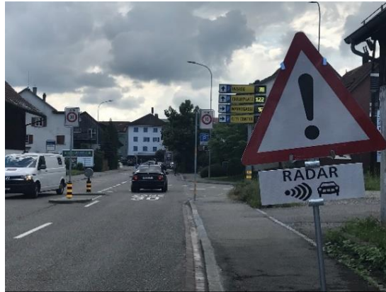
Zone-30-Tor in Wallisellenstrasse
